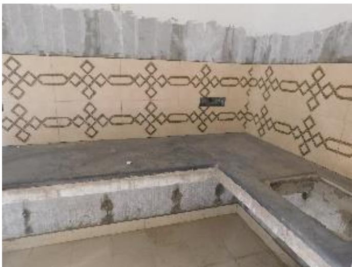
Finishing - Tiling & Kitchen Counter & False ceiling Work
