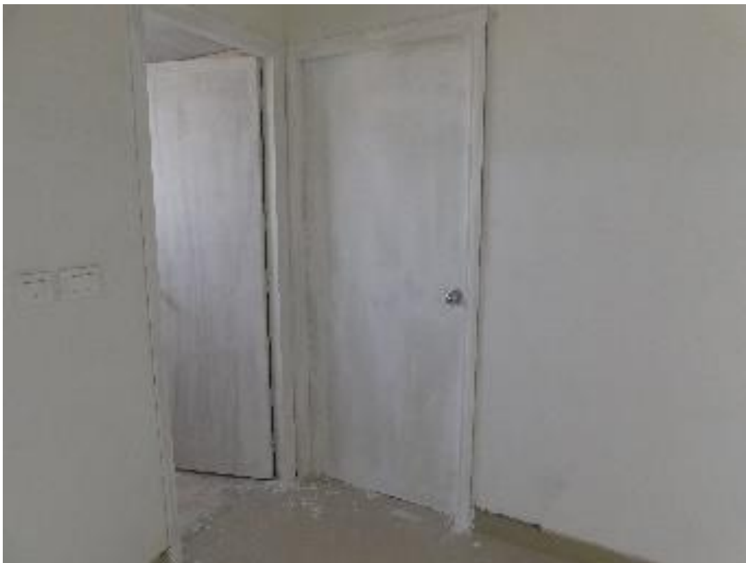
Finishing - Door Frame (Main & Internal) & Main Shutter Fixing
